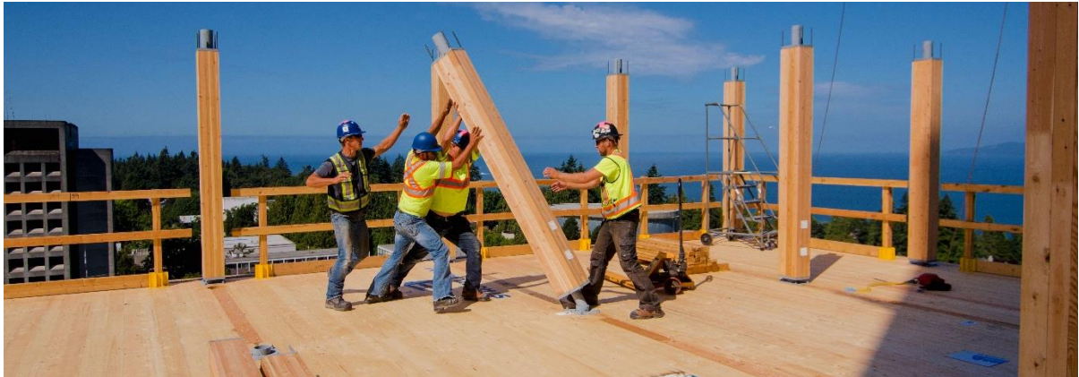
Figure 7: Crews installed columns by hand. Courtesy of Seagate Structures.
